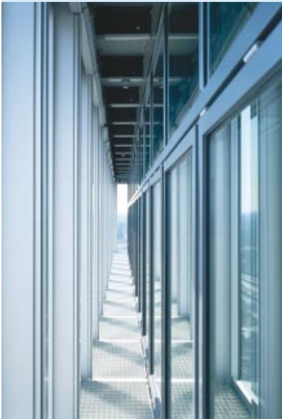
Fig. 1: In the 17-storey Fraunhofer Haus in Munich, with its large glazed areas, the cooling energy demand for concrete slab cooling can be greatly reduced by use of natural heat sinks (cool night air), as the double-glazed external facade makes natural ventilation feasible, day and night. The photo shows a view along one storey of the double-glazed facade on the south-eastern side.
