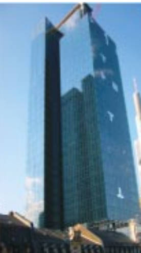
Fig. 1: The new high-rise building for the Dresdner Bank in Frankfurt am Main. The single-skin facade allows natural ventilation of the rooms. A single-skin facade is economic, not only because of the investment costs, but also because more space is available for leasing due to the thinner external walls.
