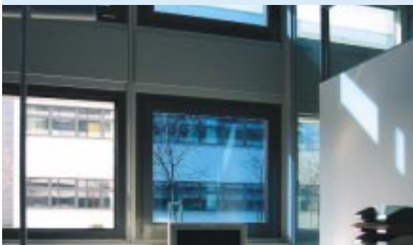
Fig. 2: View out of a Fraunhofer ISE office equipped with switchable glazing. The right-hand window has been coloured blue, the left-hand window is open. The view through the window is retained even when it is in a deeply coloured state with a total solar energy transmittance of around 15 %.
