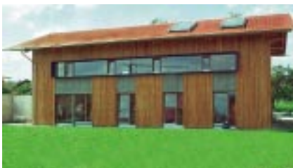
Fig. 1: Passive houses from the monitoring programme of the utility, EnBW Energie Baden-Württemberg AG. Heating system with ground-coupled heat pumps, ventilation units with heat recovery or compact ventilation units and thermal solar systems.
