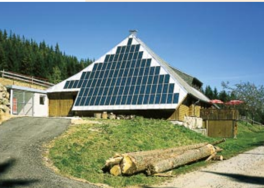
Fig. 1: The "Rappenecker Hof" with the solar generator (centre) and next to it the storage room to house the gas cylinders for the fuel cell (on the left).
