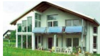
Fig. 1: Passive houses from the monitoring programme of the utility, EnBW Energie Baden-Württemberg AG. Heating system with ground-coupled heat pumps, ventilation units with heat recovery or compact ventilation units and thermal solar systems.
