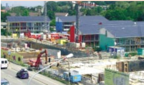
Fig. 1: In this solar settlement in Freiburg, about 40 household units with a total of 260 kWp of photovoltaics are in operation. Approximately 100 distributed inverters feed the solar electricity into the low-voltage grid.
