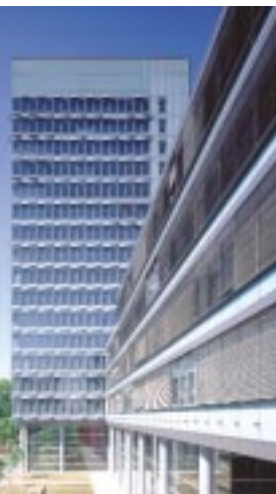
Fig. 3: The Fraunhofer Haus in Munich. The double-skin facade is part of the ventilation concept for the offices.
